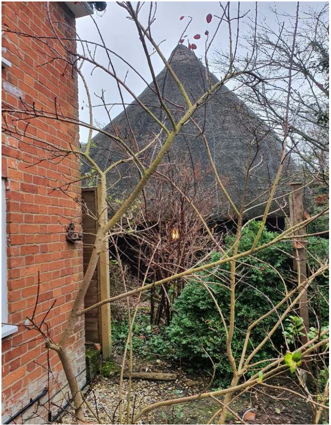
View of North Elevation of cottage at Gallants View from neighbouring property to the north
